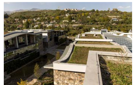
In order to preserve and increase biodiversity the roofs are mowed only twice a year.
