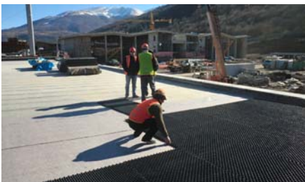
The drainage elements were laid butt jointed on all roof surfaces.
